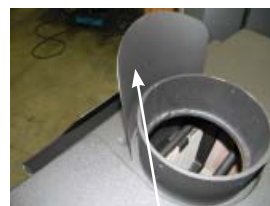
Installed Pipe Shield
