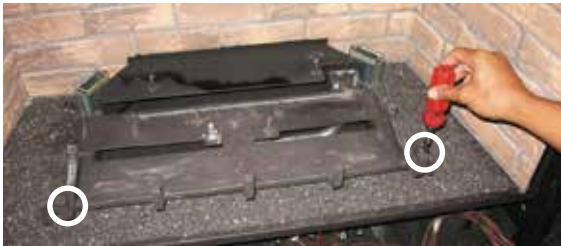
Diagram 1: Remove the left and right screws.
