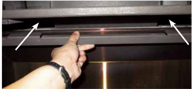
Top panel bracket shown installed with Stainless Steel Panels
