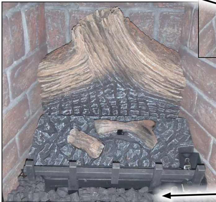
Figure 37. Coal Nuggets Installation.
