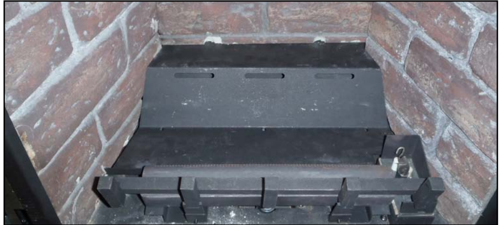
Figure 35. Empty firebox with grate and locator pins.
