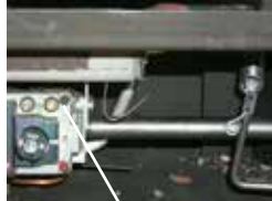
Adjustment wire: Push to close or pull to open aeration cap.
