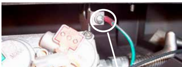
Green ground wire
