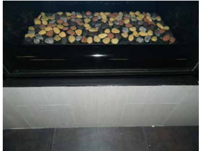
Figure 102: Completed Trim install
