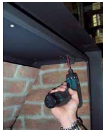
Figure 80: Right Side Brick Panel
