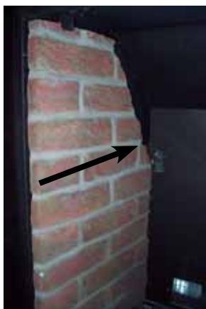
Figure 78: Left Brick Panel
