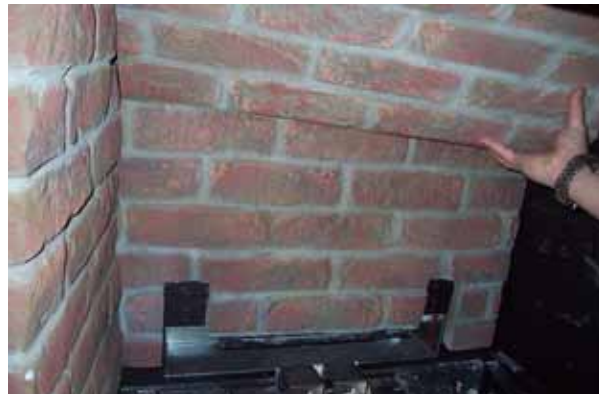
Figure 79: Upper Back Brick Panel
