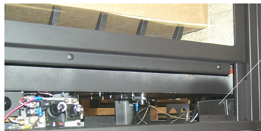
Remove cover to access Terminal Block
