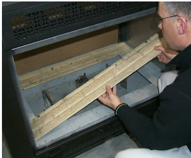
Remove the 2 Long Base Brick Panels
