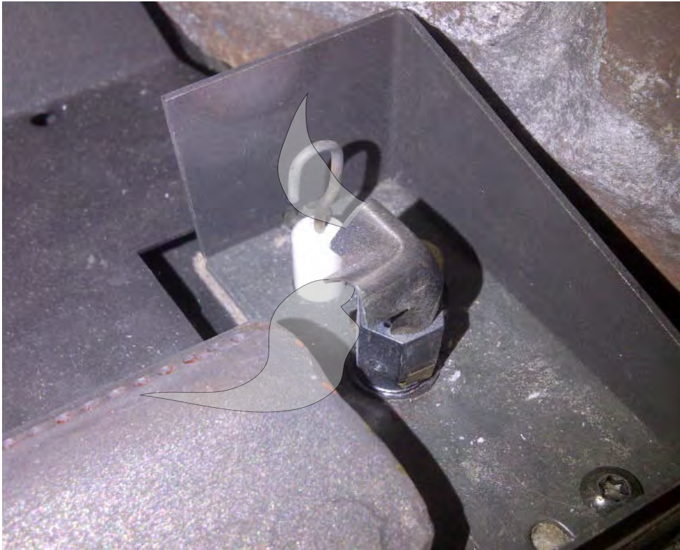
Figure 21. Correct Burner & Pilot Shield Placement
