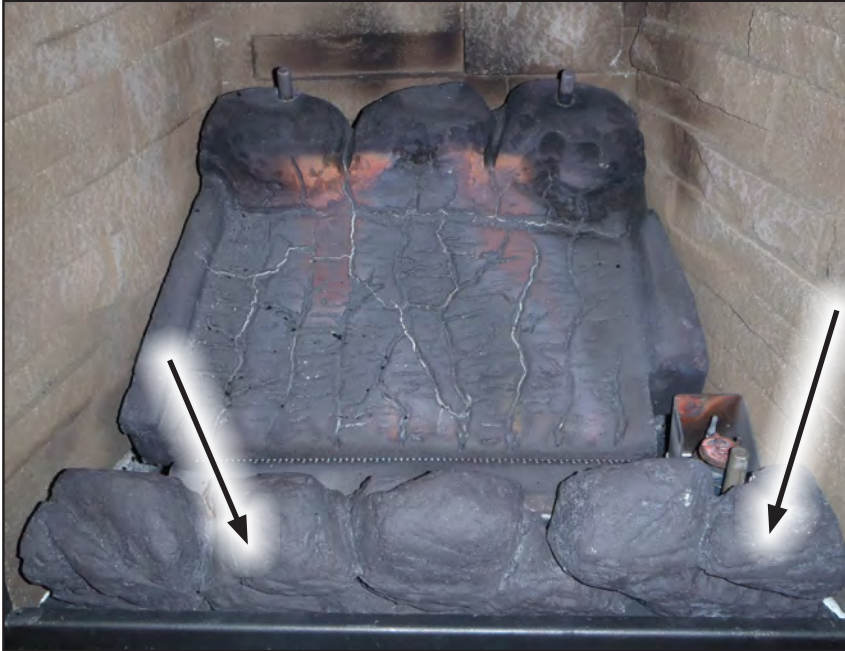
Figure 58. Second Stage Coal Set Installation.
