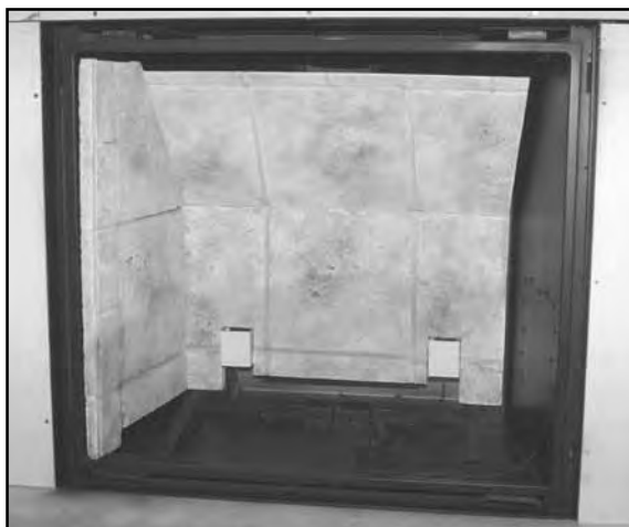
Figure 65: Top Firebox Liner Panel in Place.
