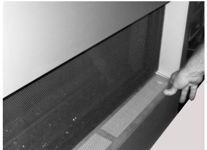
STEP 8: Tilt the Panel down to rest on the face support.
