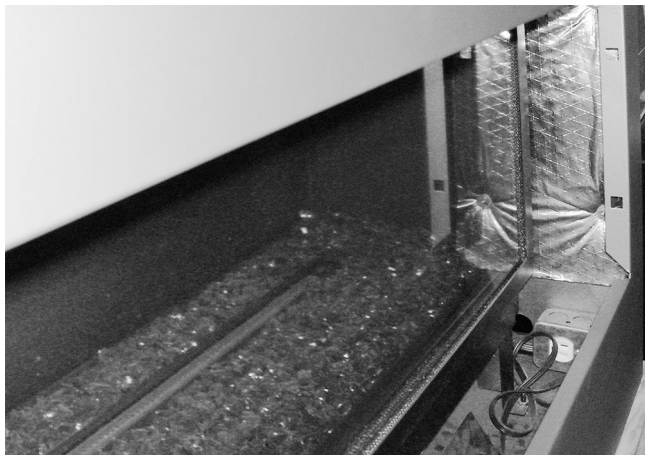
STEP 1: Remove front air panel and both side panels.
