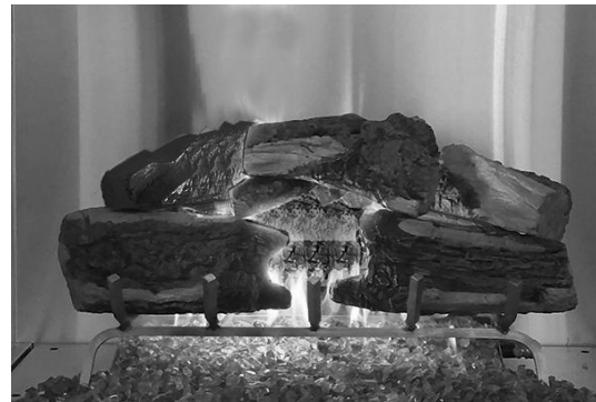
Figure 9 - Incorrect Burner Flame Pattern caused by port blockage
