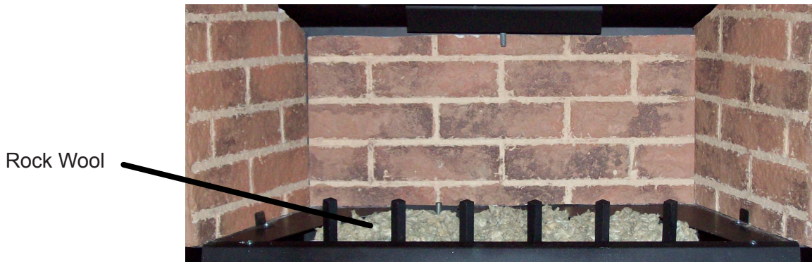
Figure 16 - Rock Wool Placement
