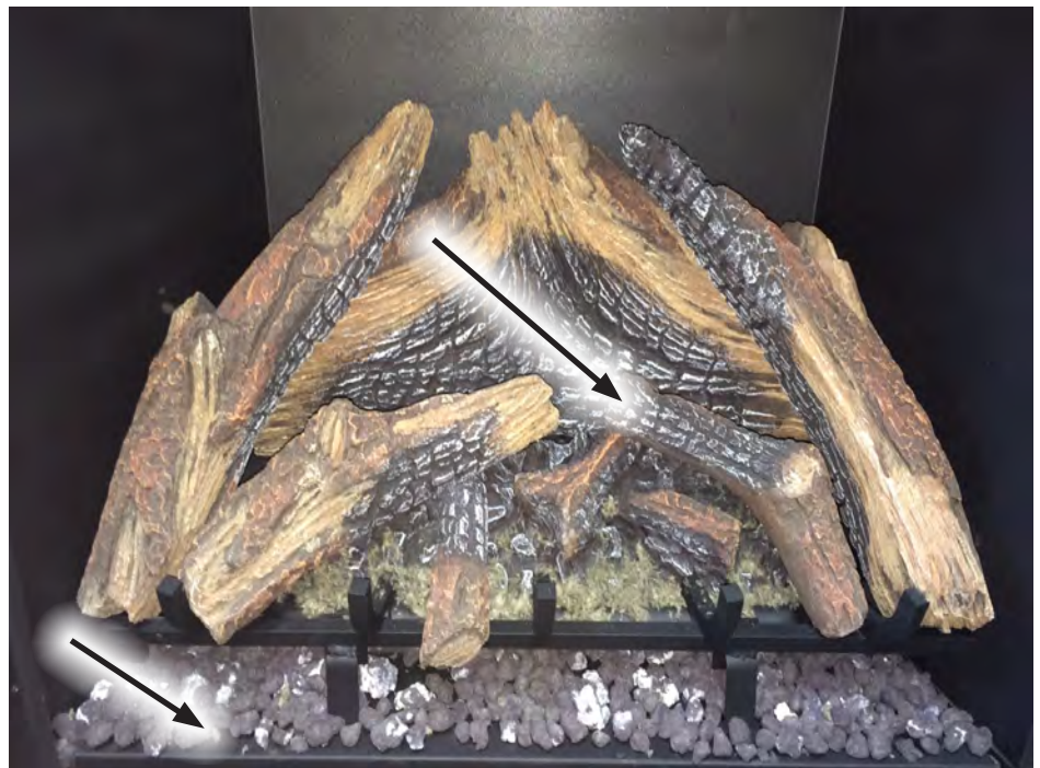
Figure 45. Fourth Stage Log Set Installation
