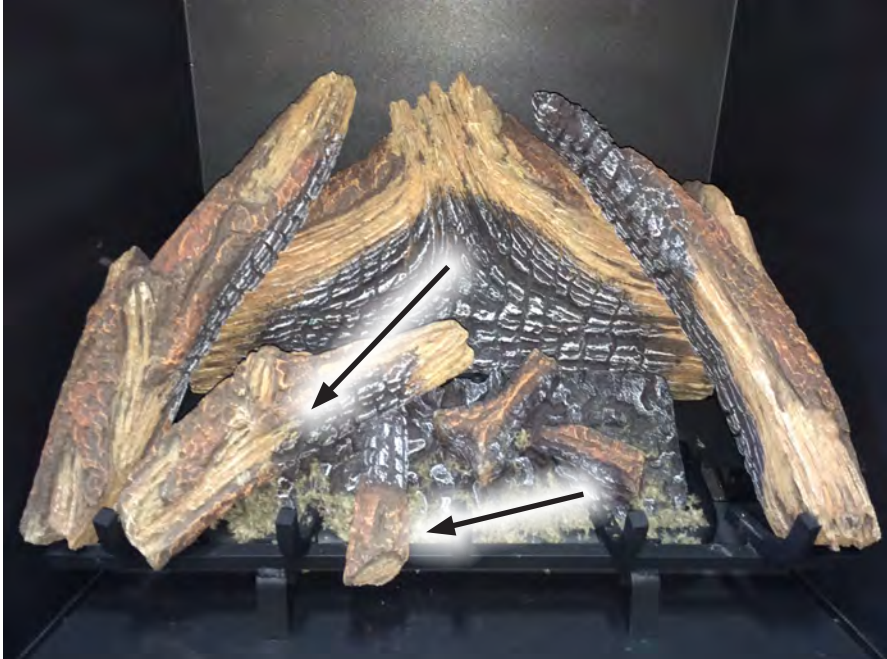
Figure 44. Third Stage Log Set Installation
