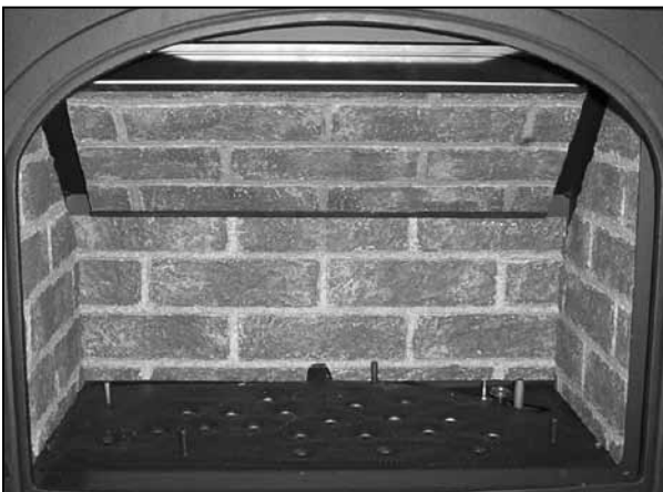
Figure 65: Side brick panels in place.
