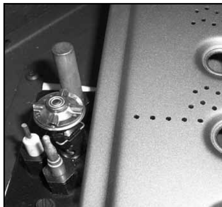
Figure 13. Ignitor assembly beside the burner.
