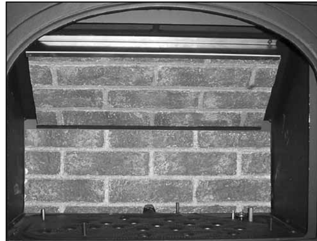
Figure 64: Back brick panel in place.
