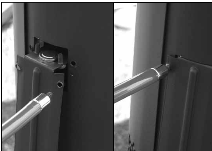
Figure 49: Spill switch installation.
