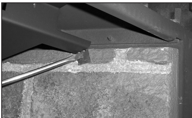
Figure 51. Top Tab For Right Panel.
