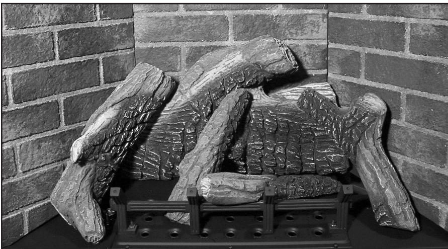
Figure 46. Fifth Stage Log Set Installation.
