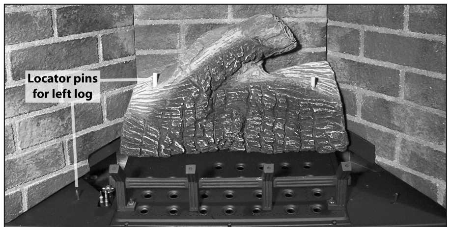
Figure 42. First Stage Log Set Installation.
