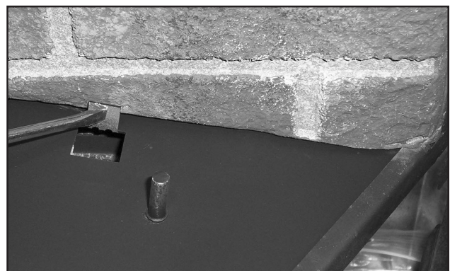
Figure 52. Bottom Tab For Right Panel.
