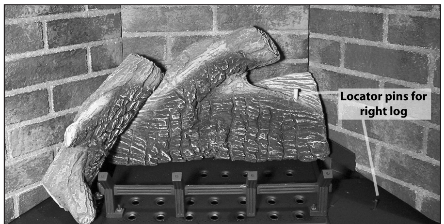
Figure 43. Second Stage Log Set Installation.
