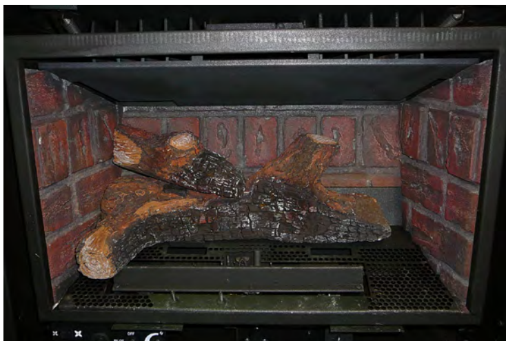
Figure 68. Second Stage Log Set Installation.
