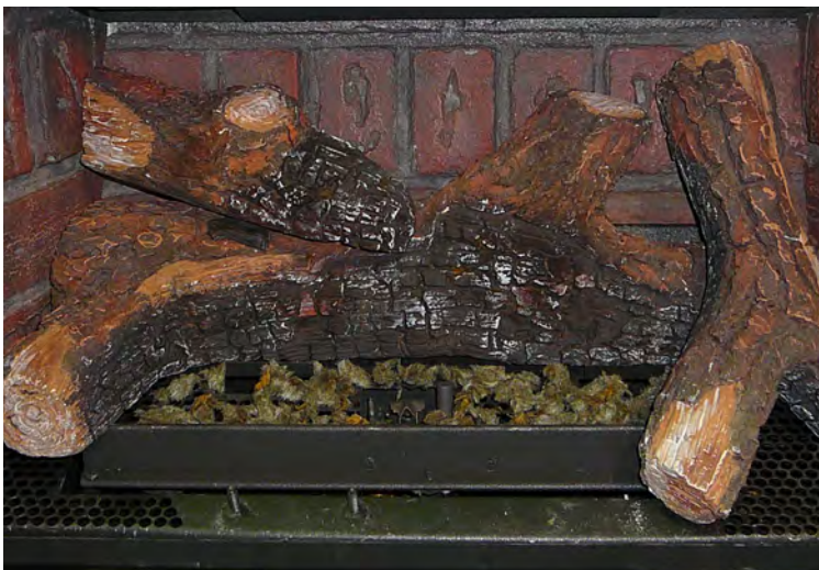
Figure 71. Fifth Stage Log Set Installation.
