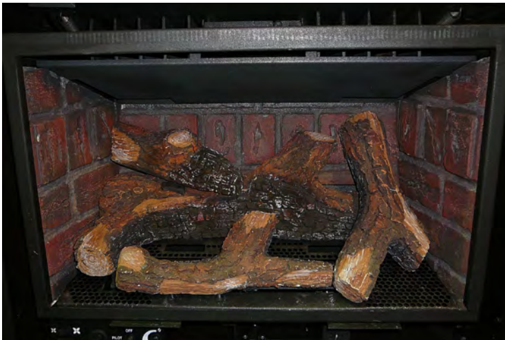
Figure 70. Fourth Stage Log Set Installation.
