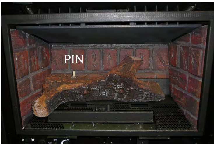
Figure 67. First Stage Log Set Installation.
