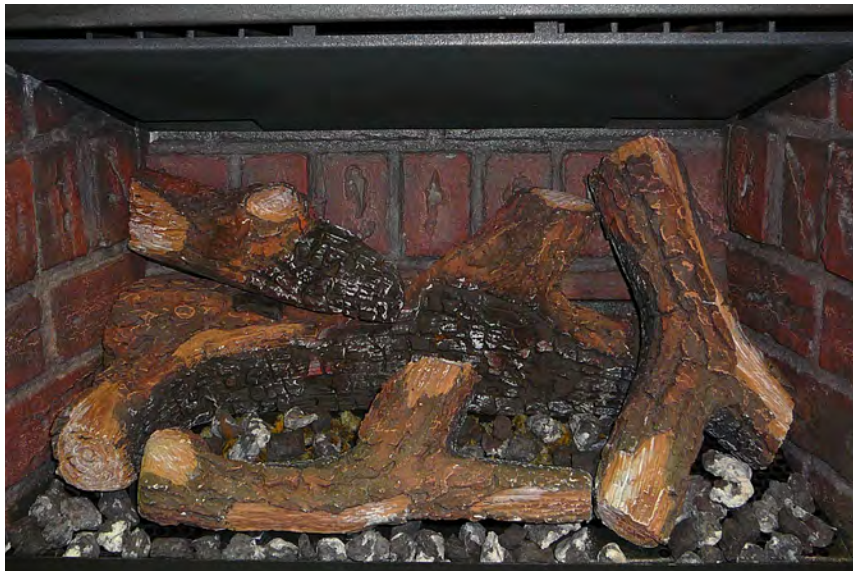
Figure 72. Log Set and Ember Installation.
