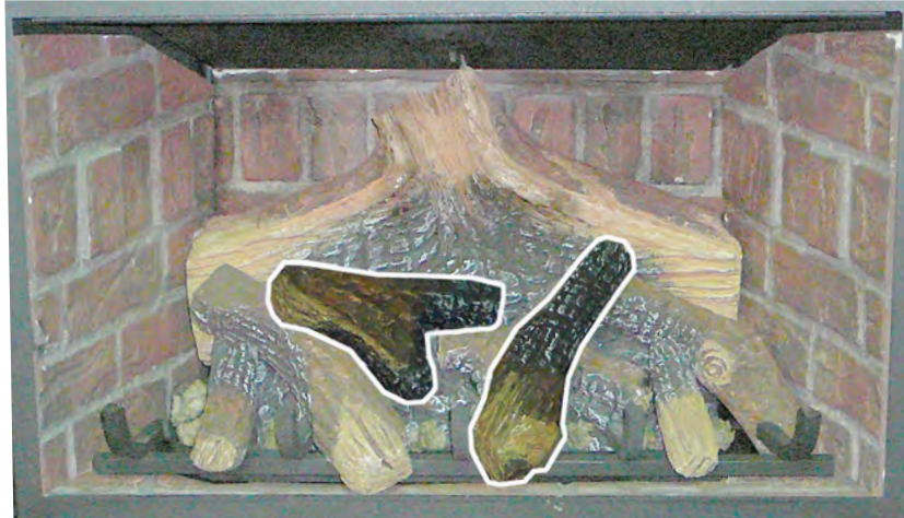
Figure 69: Seventh Stage Log Set Installation.
