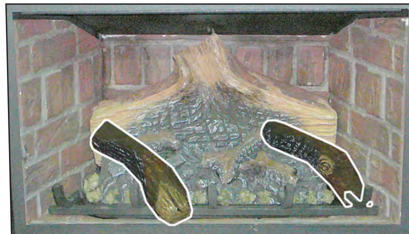
Figure 55: Fifth Stage Log Set Installation.
