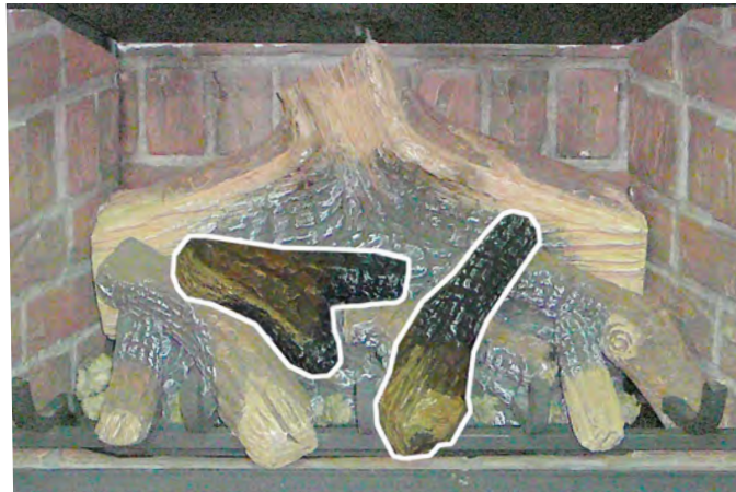
Figure 65: Seventh Stage Log Set Installation.
