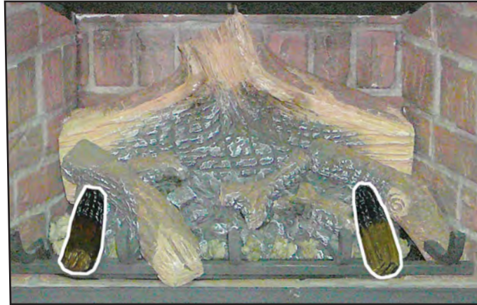
Figure 64: Sixth Stage Log Set Installation.
