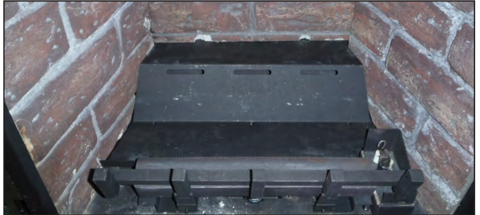
Figure 56. Empty firebox with grate and locator pins.
