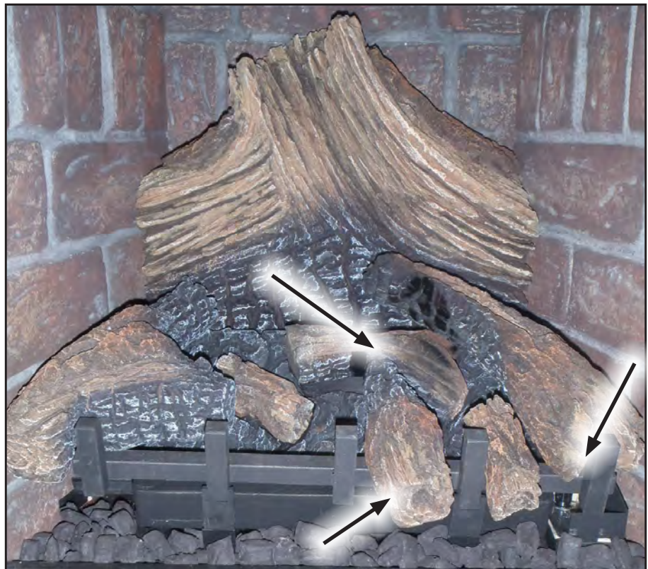
Figure 60. Fourth Stage Log Set Installation.
