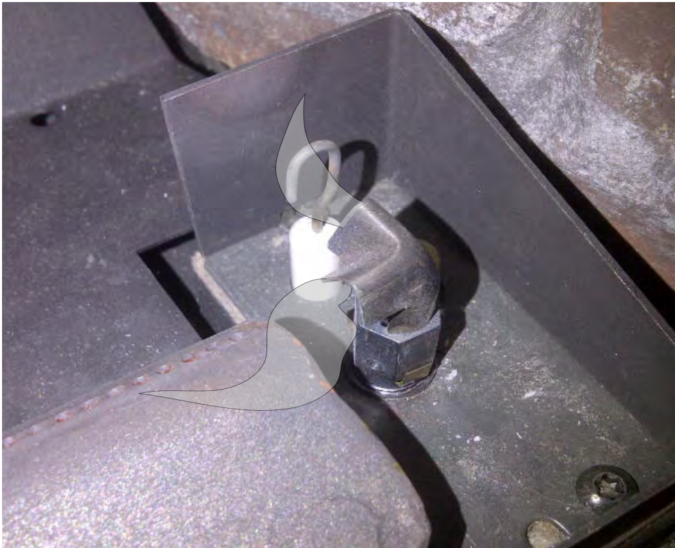
Figure 21. Correct Burner & Pilot Shield Placement
