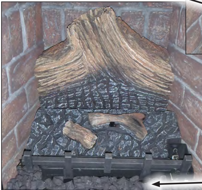
Figure 58. Coal Nuggets Installation.
