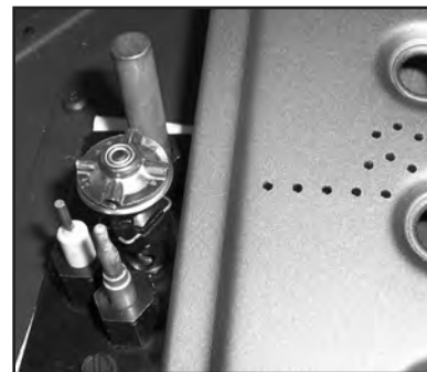
Figure 15: Burner to pilot hood relationship.
