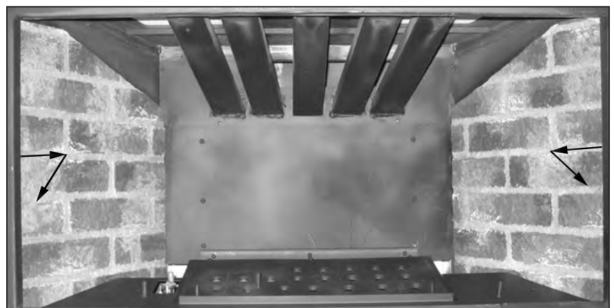
Figure 40: Brick Panel Installation.
