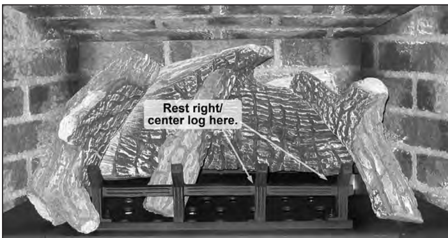
Figure 33. Second Stage Log Set Installation.
