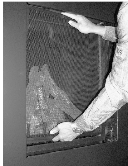
STEP 3: Lift the Safety Screen up so the tabs slide over the mounting bolts on the glass frame.
