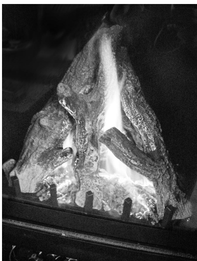
Figure 53 - Burner Flame Appearance
