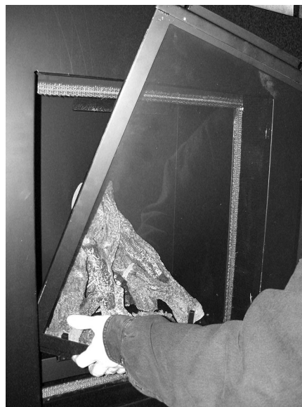
Figure 36 - Removing Glass Frame
