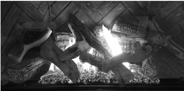
Figure 53 - Burner Flame Appearance
