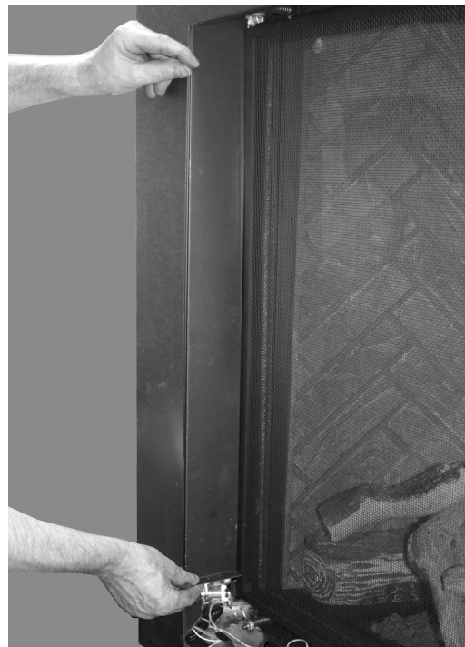
STEP 2: Match up the tabs in the panel with the slots in the face and slide downward. Make sure the Side Panel is secured properly. Repeat with opposite side panel.
