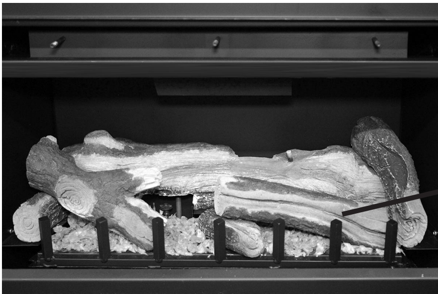
Figure 22 - Installing Right Upper Log #6
