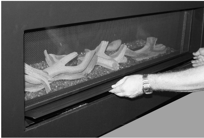
STEP 7: Angle the Air Front Panel beneath the bottom of the screen. Support the Air panel on the left and right Side Panels.
