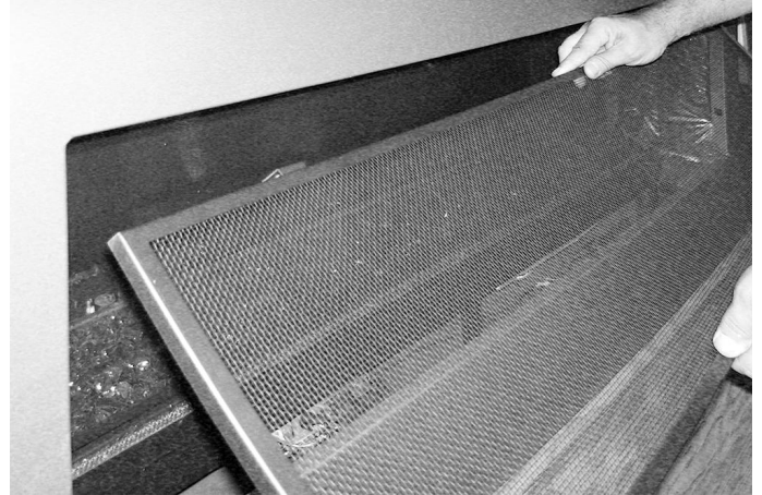
STEP 2: Angle the safety screen as shown on the picture and carefully bring into the fireplace opening.
